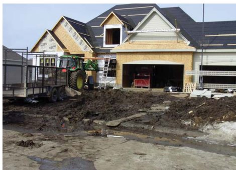
The lack of sediment controls on this site could result in polluted water and compliance violations.
