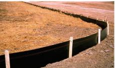
the fence. Remove sediment deposits as necessary to provide adequate storage volume and reduce pressure on the fence.
