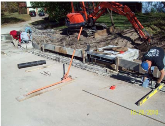
Inlet being installed on Brampton Court.
