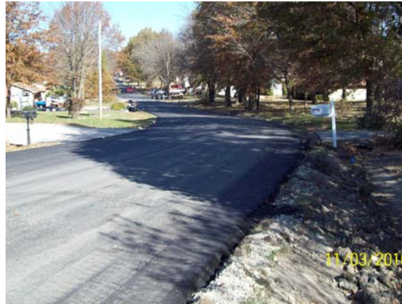
Completed asphalt overlay on Broadview Court in an area without concrete curb and gutter.
