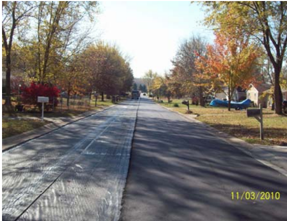
Installation of asphalt overlay with paving fabric between concrete curb and gutter
