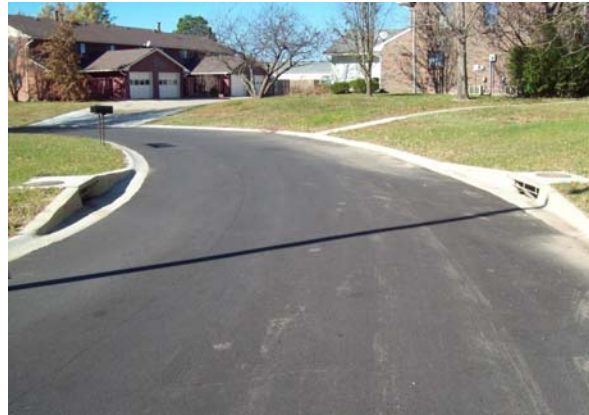
New storm water inlets on Pinehurst Drive.
