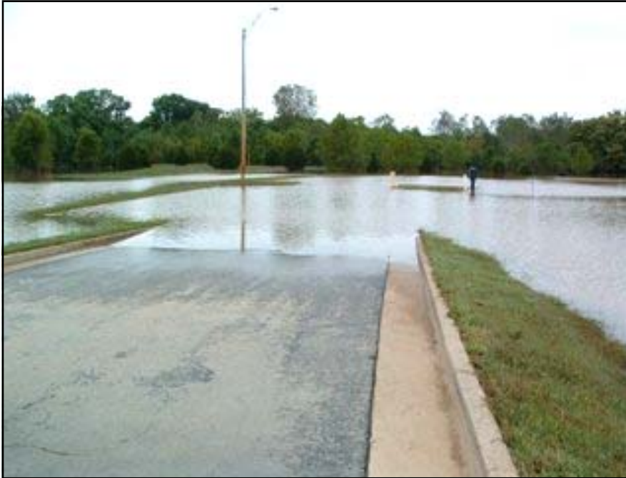
MKT Trailhead Parking Lot
