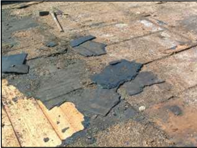
Roof Deterioration
