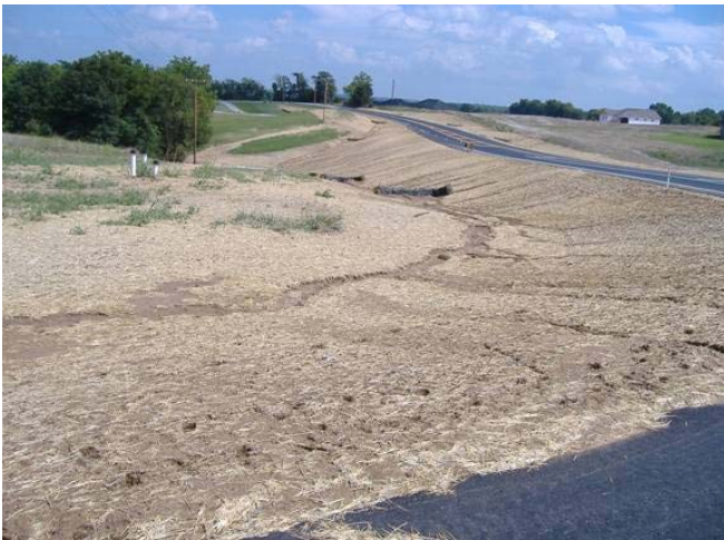
Ditching along Route K
