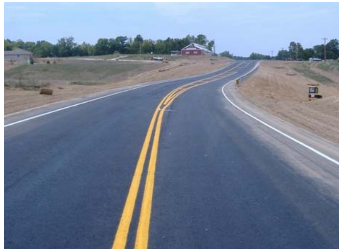
Route K Completed
