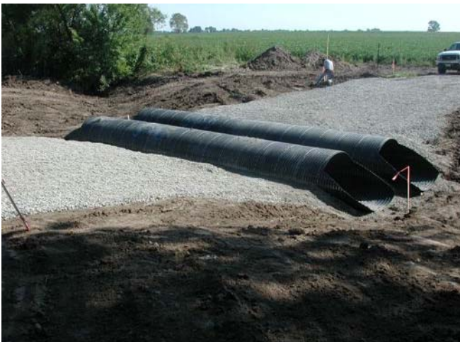
Green Road Low Water Crossing During Construction Phase
