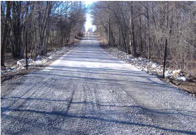
Thomas Hill Road Completed
