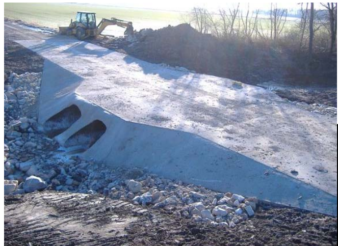
Green Road Low Water Crossing During Construction Phase
