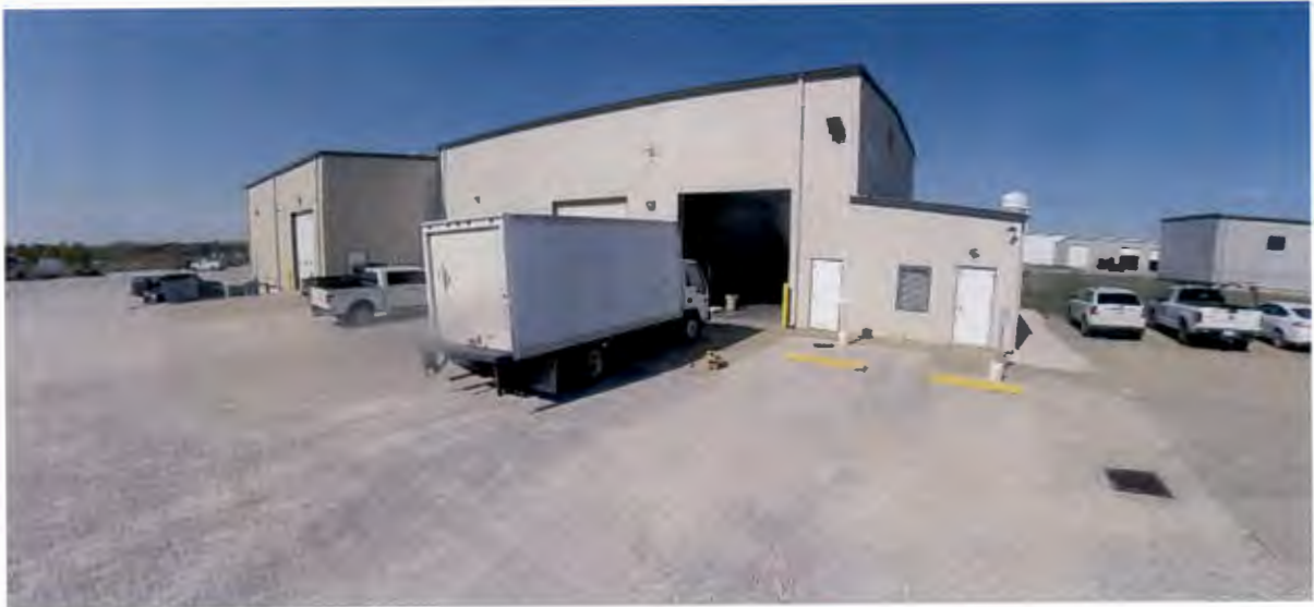
Figure 1 – Existing western building
