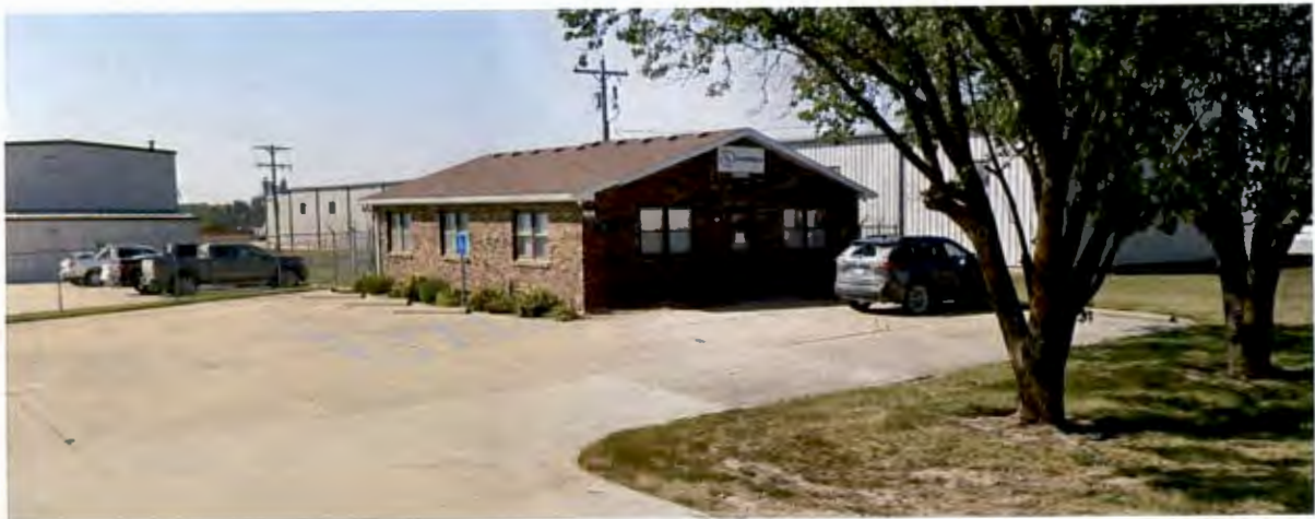
Figure 2 – Existing eastern building
