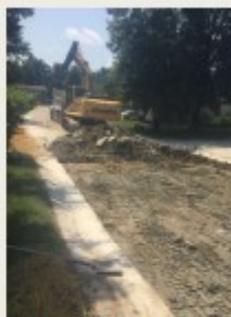
Step 3: Pavement Removal/Excavation
