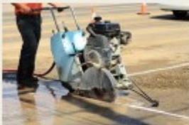
Step 1: Saw Cut for Curb Repair
