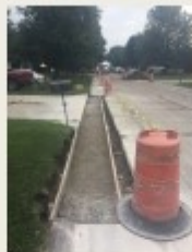
Step 2: Curb and Gutter Repair
