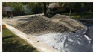
Step 4: Fabric & Base Rock Installation
