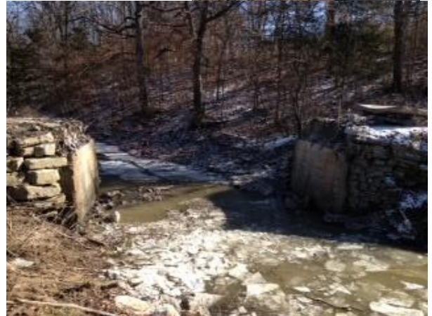
Old abutment with bridge deck removed
