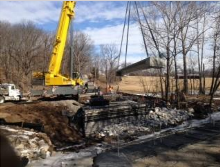
Placing girders Rustic Rd Bridge
