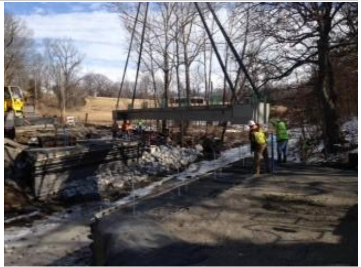
Placing girders Rustic Rd Bridge
