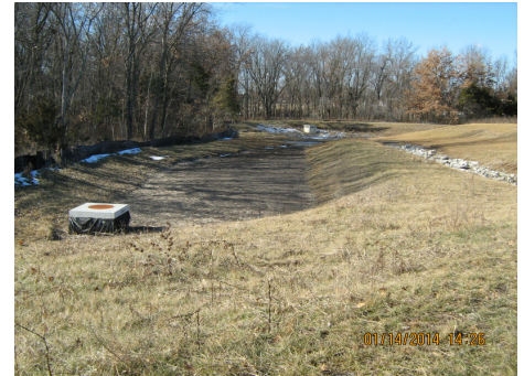
Bio retention cell at Meyer Industrial Dr. Bioretention cells are used to treat polluted stormwater runoff from impervious surfaces. This photo is winter dormant.
