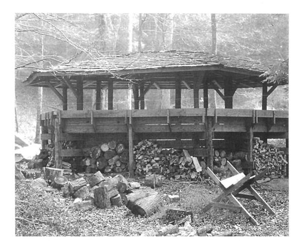
This design is from the Tremont Insititute located in the Great Smoky Mountains National Park. The design allows amphitheater seating around a central fire pit. The seating is protected from the elements, while smoke exits the structure through a hole in the center of the roof. Fire wood can be stored under the seating area.
