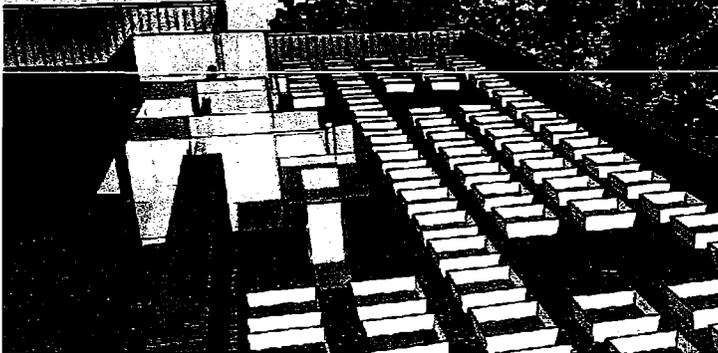
Geosyntec is helping to implement low impact development design techniques, such as this blue roof, to minimize combined sewer overflows in New York City.
