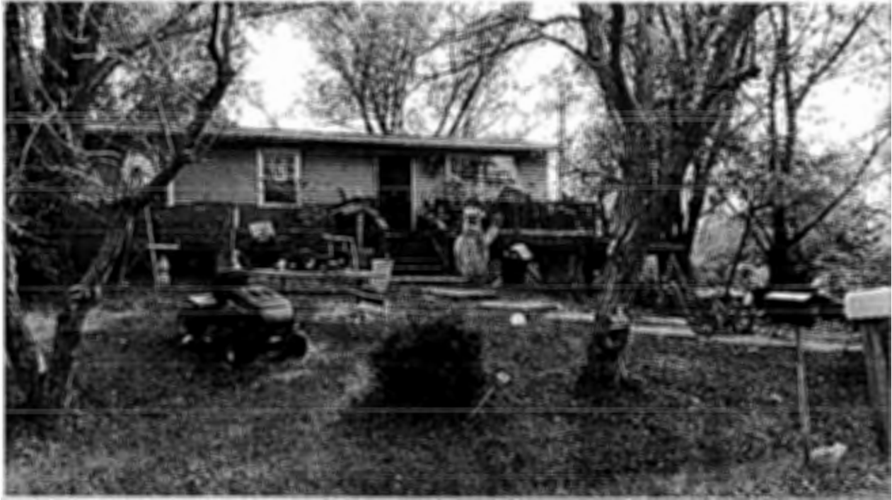
Photographs taken 10/25/16 @ ~ 3:00 pm 440 E. Clearview Drive
