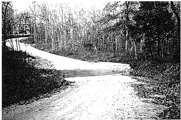
Ginn Lane South Crossing
