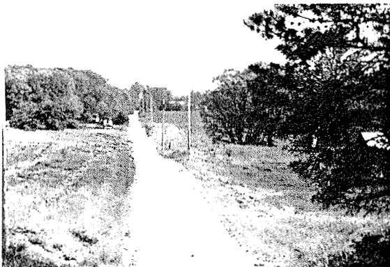
Caruthers Road -Before improvement (Widened and fill work done)
