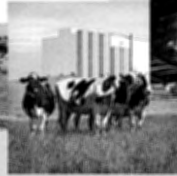
2013 Plant expansion and Cold Storage Facility construction
