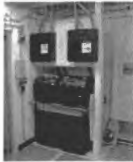
Uninterruptible Power Supply(s)
