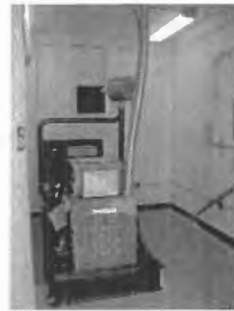
Indoor Generator Room (optional)
